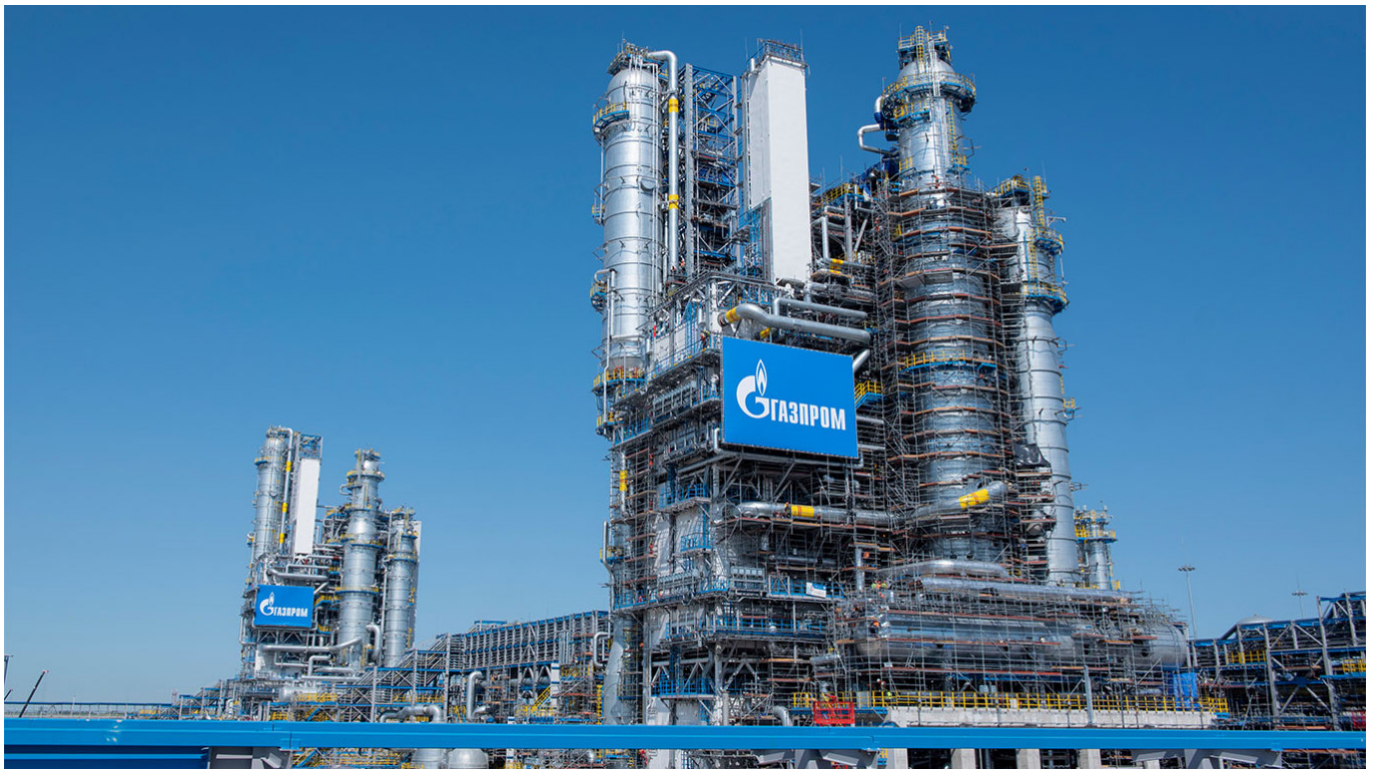
Amursk gas processing plant. Gazprom
