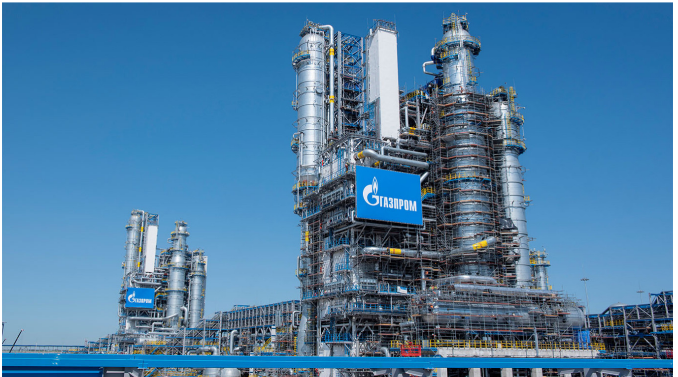
Amursk gas processing plant. Gazprom
