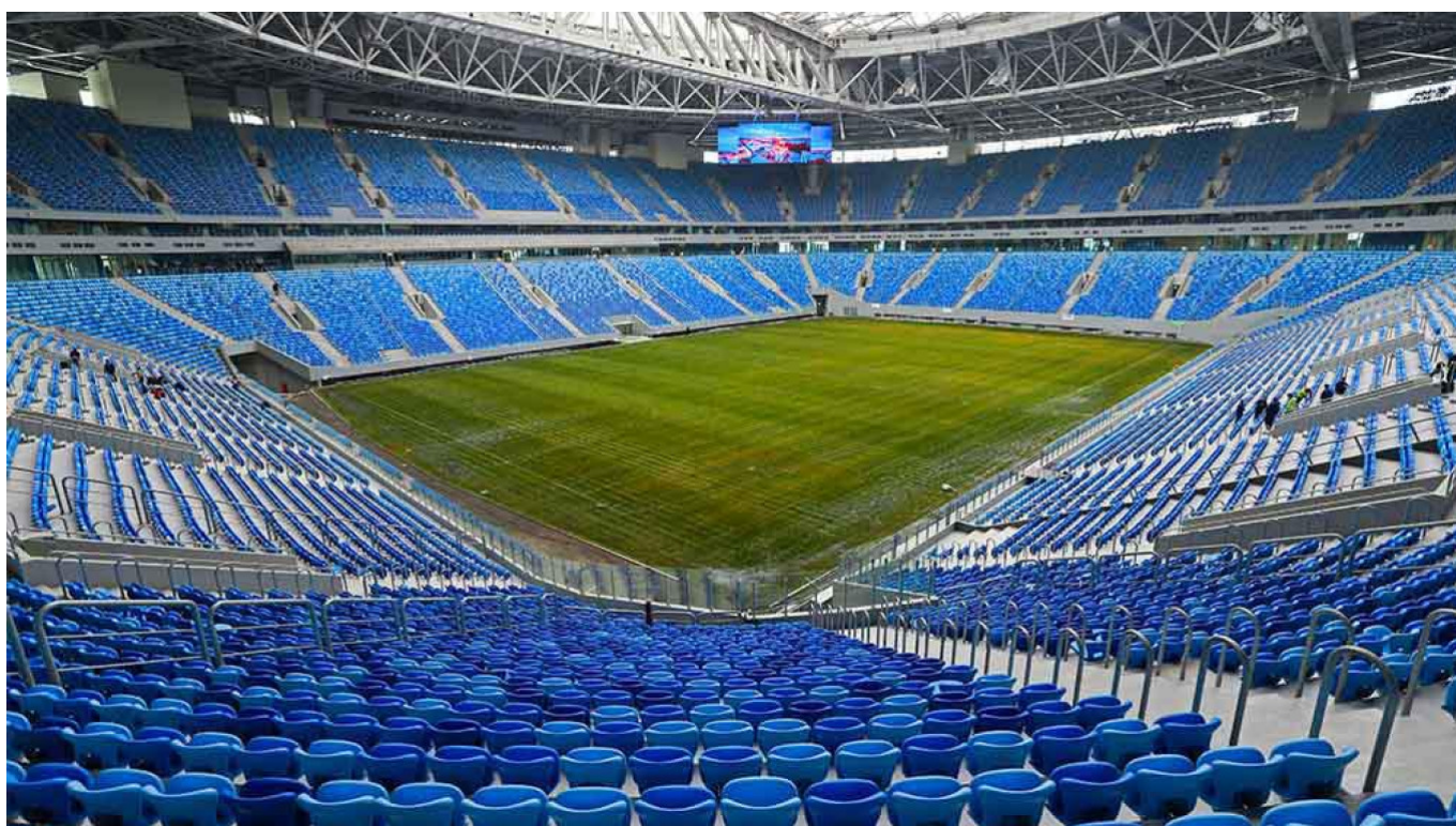
Zenit Arena Stadium in St. Petersburg (Alexander Demyanchuk / TASS)
