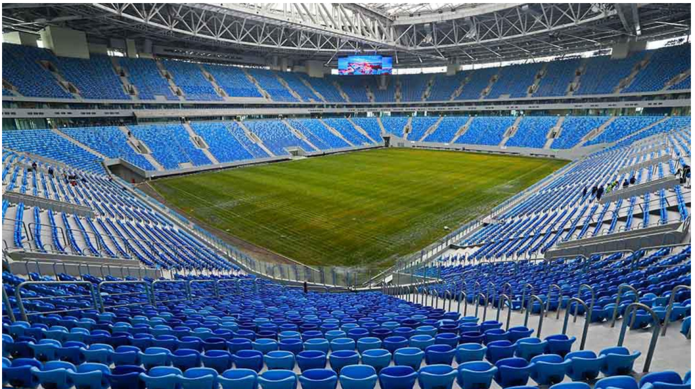
Zenit Arena Stadium in St. Petersburg (Alexander Demyanchuk / TASS)
