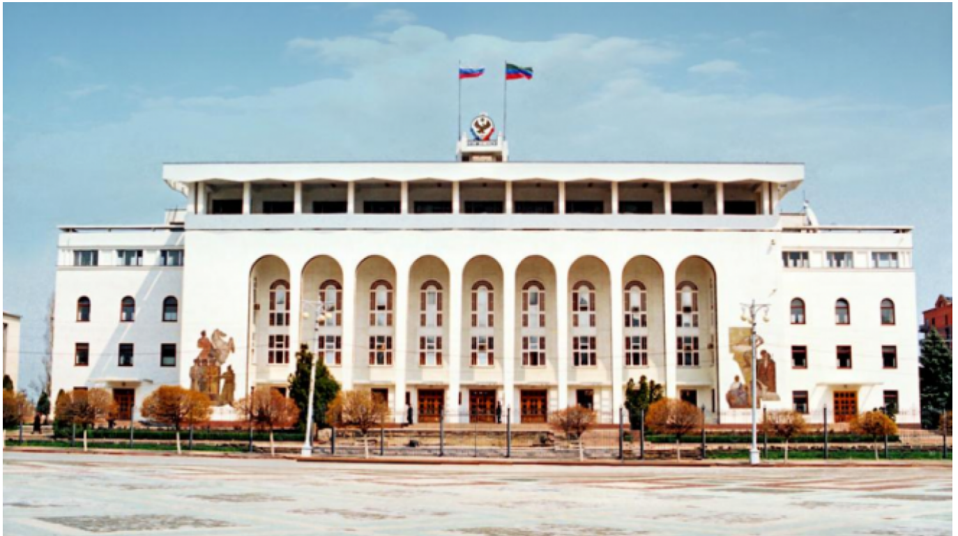
The Government building of the Republic of Dagestan
