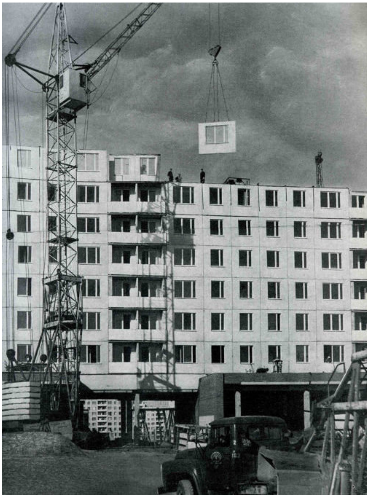
Construction of panel housing on Ulitsa Mitlukho-Maklaya. (ag84 / oldmos.ru)
